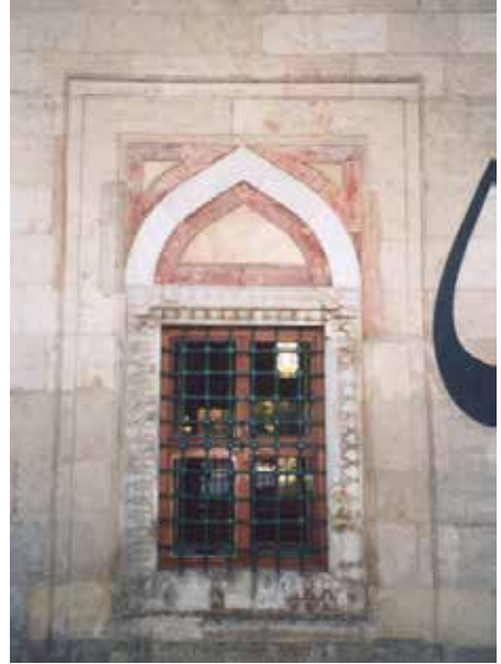
Image 10. Edirne Eski Mosque, north facade, window
