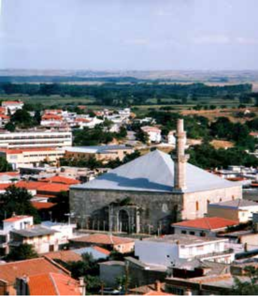
Image 1. Didymóteicho Çelebi Mehmed Mosque, north-west facade
