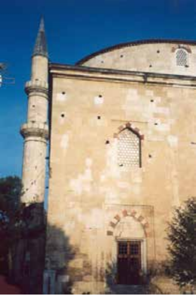
Image 9. Edirne Eski Mosque, south facade
