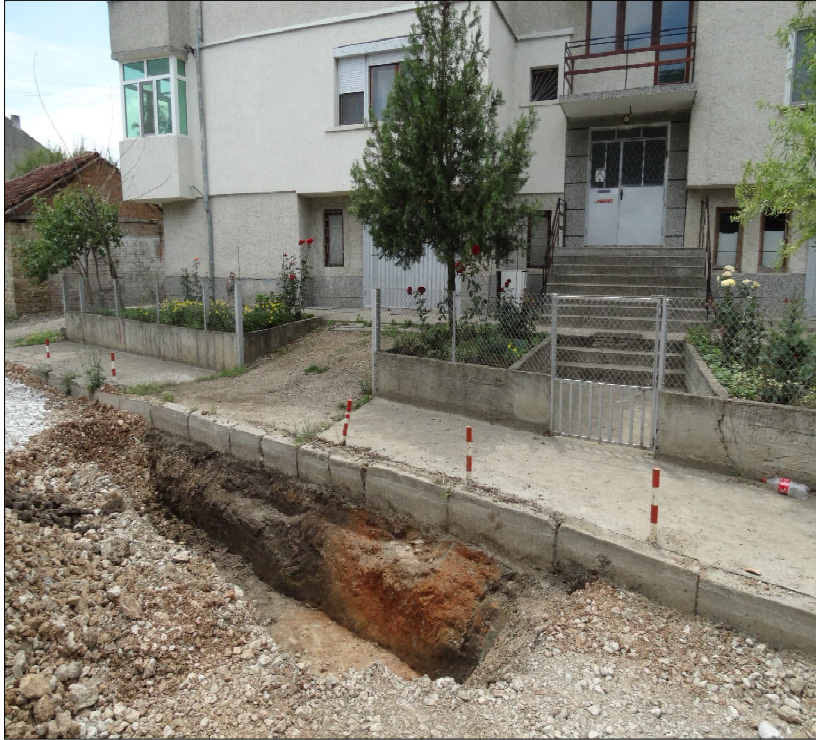
Figure 25 – Kiln No. 10 – initial phase of excavation (K. Chakarov)
